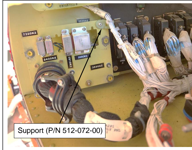
Figure 3.60 Wire Support Installation
