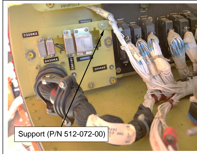
Figure 3.60 Wire Support Installation
